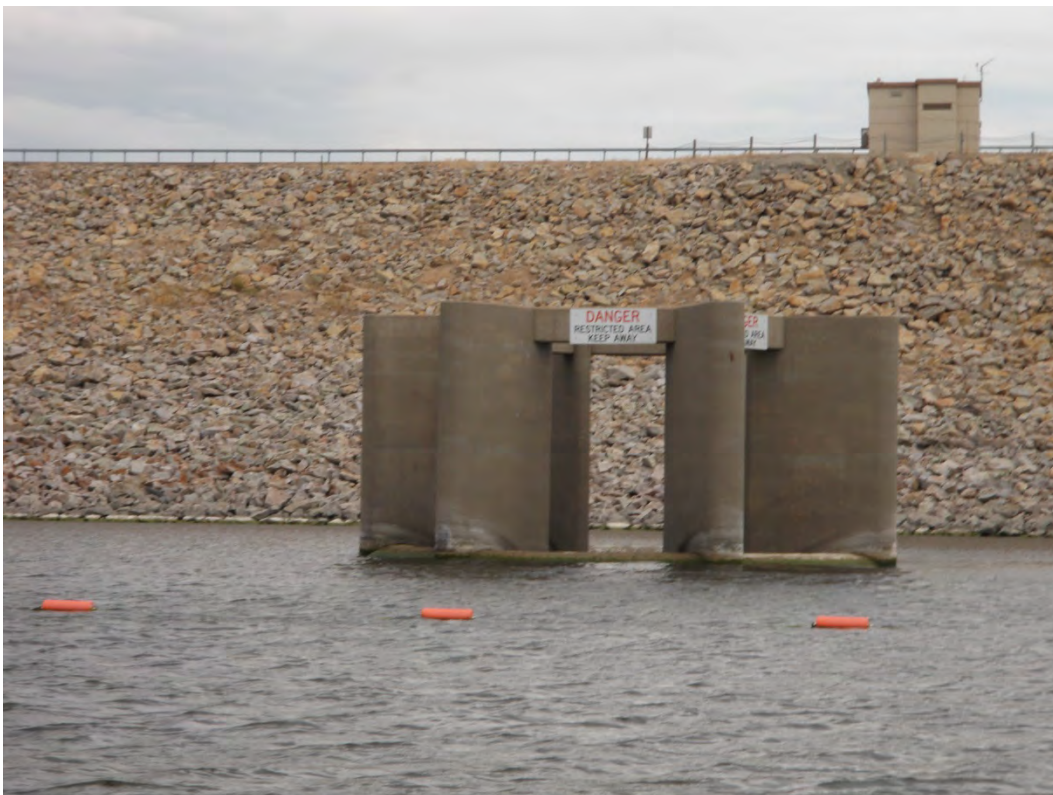
Figure 3 - Uncontrolled concrete glory hole spillway at water surface elevation 2,064.
