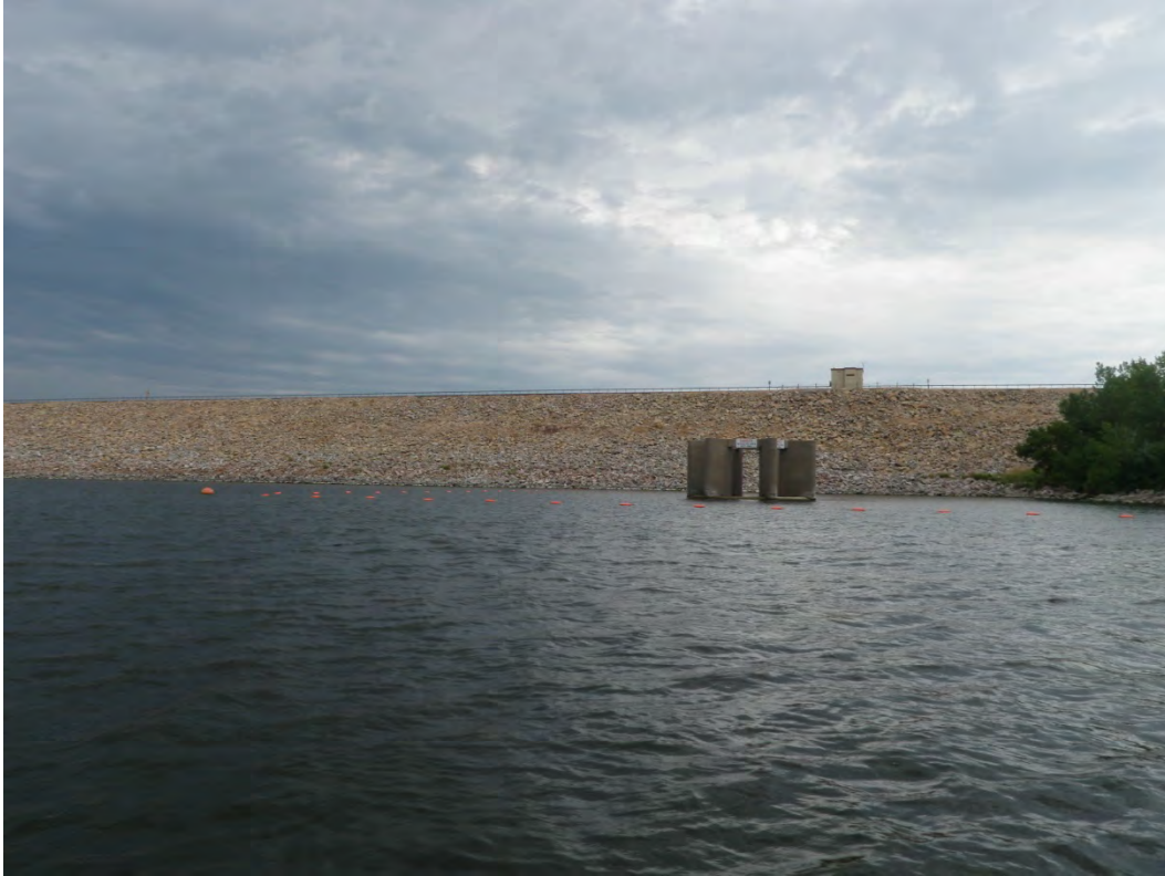
Figure 2 - Heart Butte Dam and uncontrolled concrete glory hole spillway.
